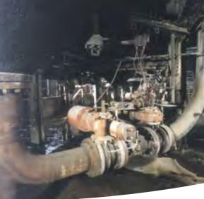
nitrogen tested. All oxygen service assemblies are then polyethylene packaged. While other materials are available upon request, 316 stainless steel is the standard material for oxygen service.
