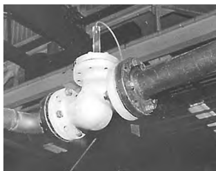
Figure 8 Size 4 Class 600 90° bonnet piston lift check valve with two upstream elbows (out of plane). This arrangement produces swirl as shown in Figure 7.
